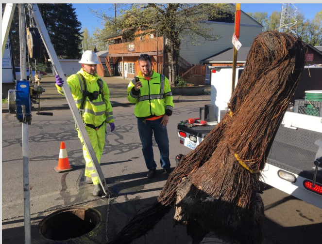
A 13ft, 200lb root-ball from a nearby street-tree removed from a manhole at Washougal River Road & A Street. The root was discovered during a routine manhole inspection.
