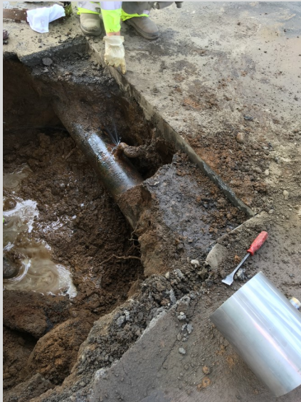
Staff repairing a water main leak.
