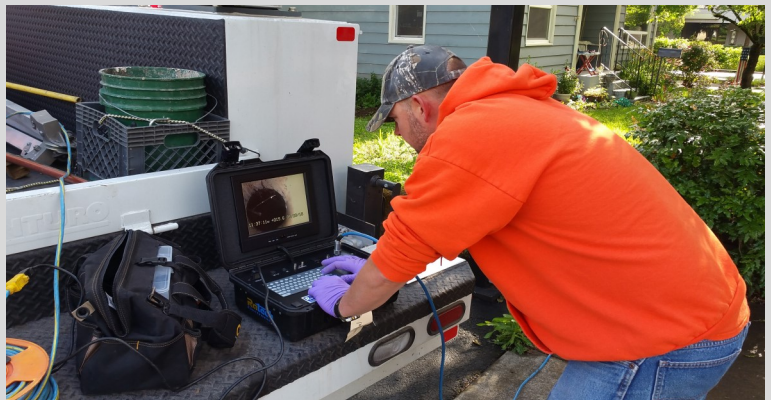
Staff using inspection camera to look at a customers line.
