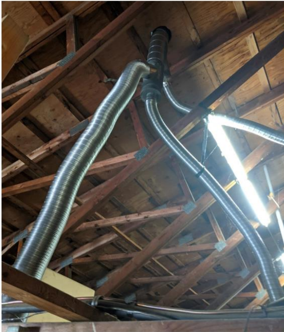
Figure 4.7. Building A Exhaust Connections
