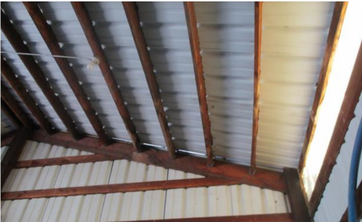
Figure 2.9. Gap at Edge of Roof
