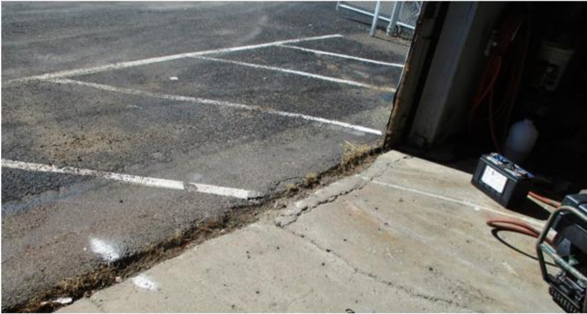
Figure 2.2. Example of Transition Between Asphalt and Concrete
