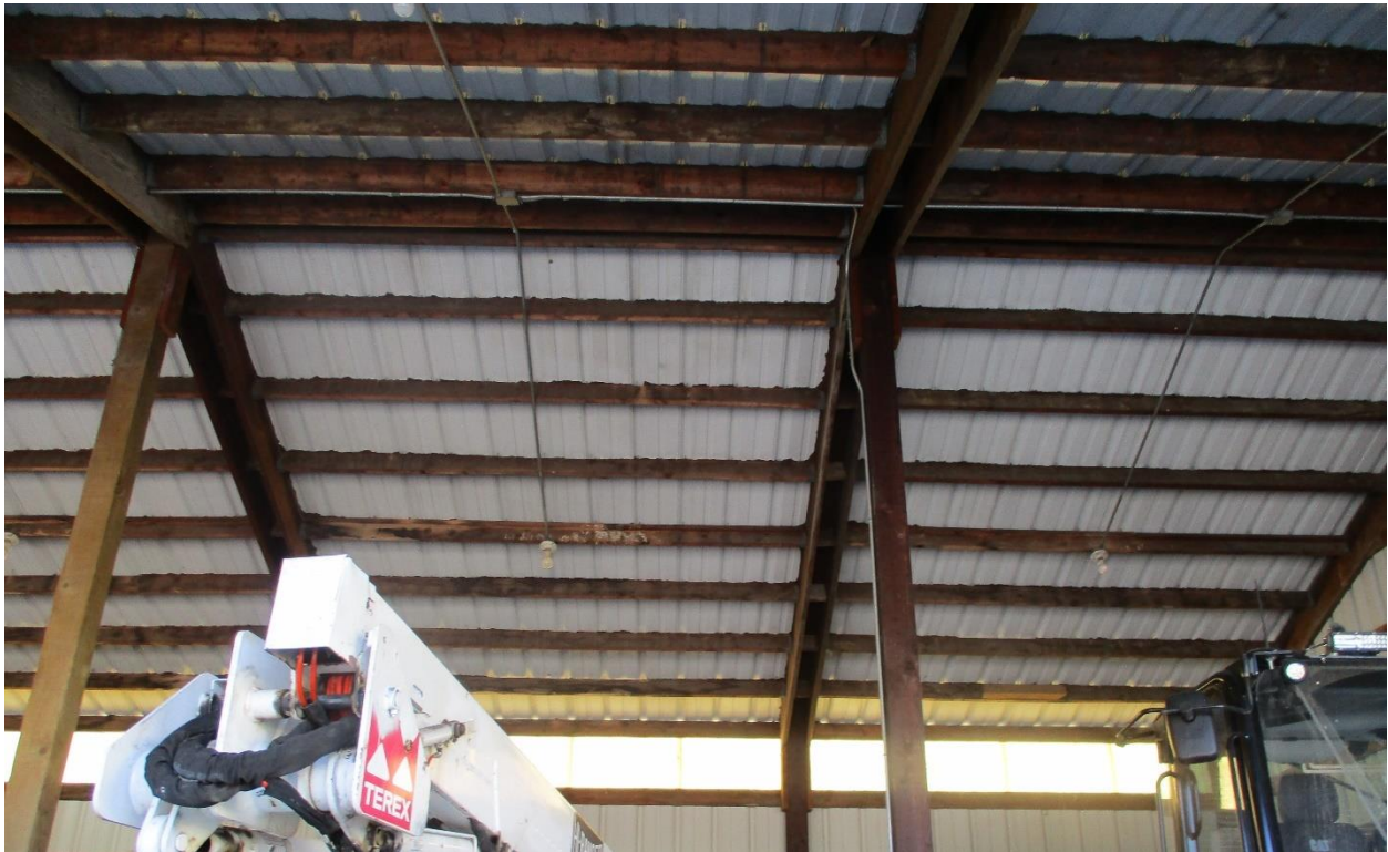
Figure 2.9. Gap at Edge of Roof
