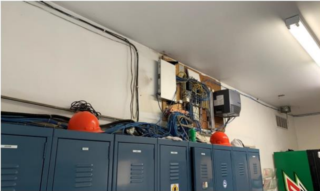
Figure 3.2. Exposed Communication Equipment
