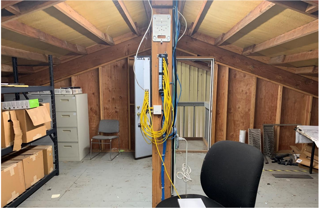
Figure 3.7. Communication Cables in Loft Space
