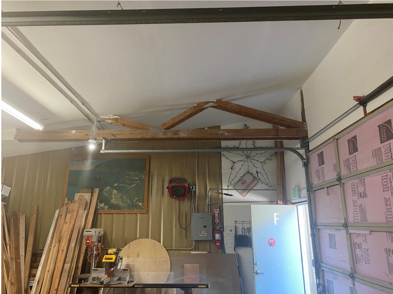
Figure 2.20. Roof Structure Hidden with Drywall
