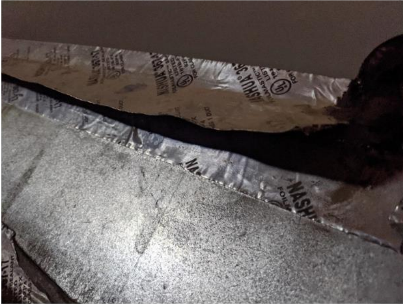
Figure 4.3. Building A Air Leak
