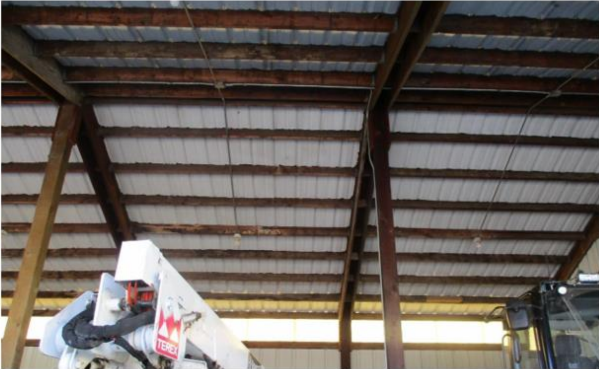
Figure 2.9. Gap at Edge of Roof
