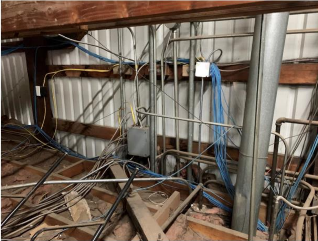
Figure 3.4. Communication Cables in Attic
