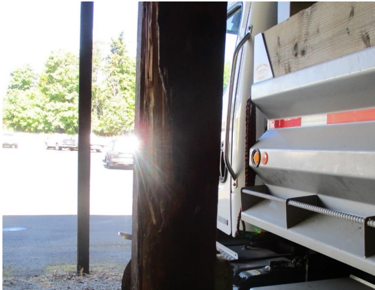
Figure 2.11. Column Damage
