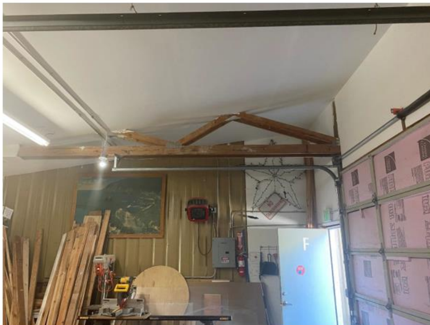
Figure 2.20. Roof Structure Hidden with Drywall
