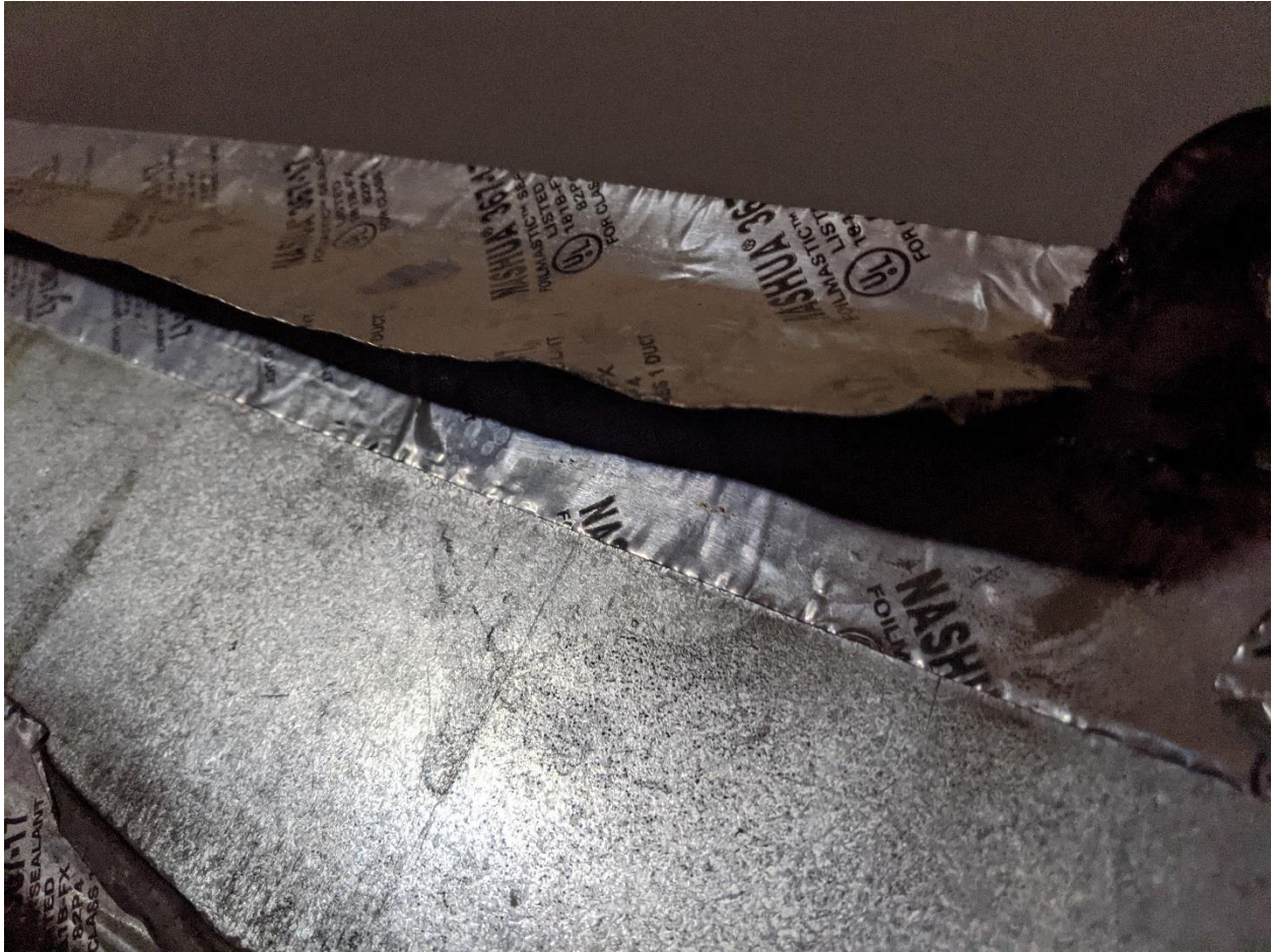
Figure 4.3. Building A Air Leak
