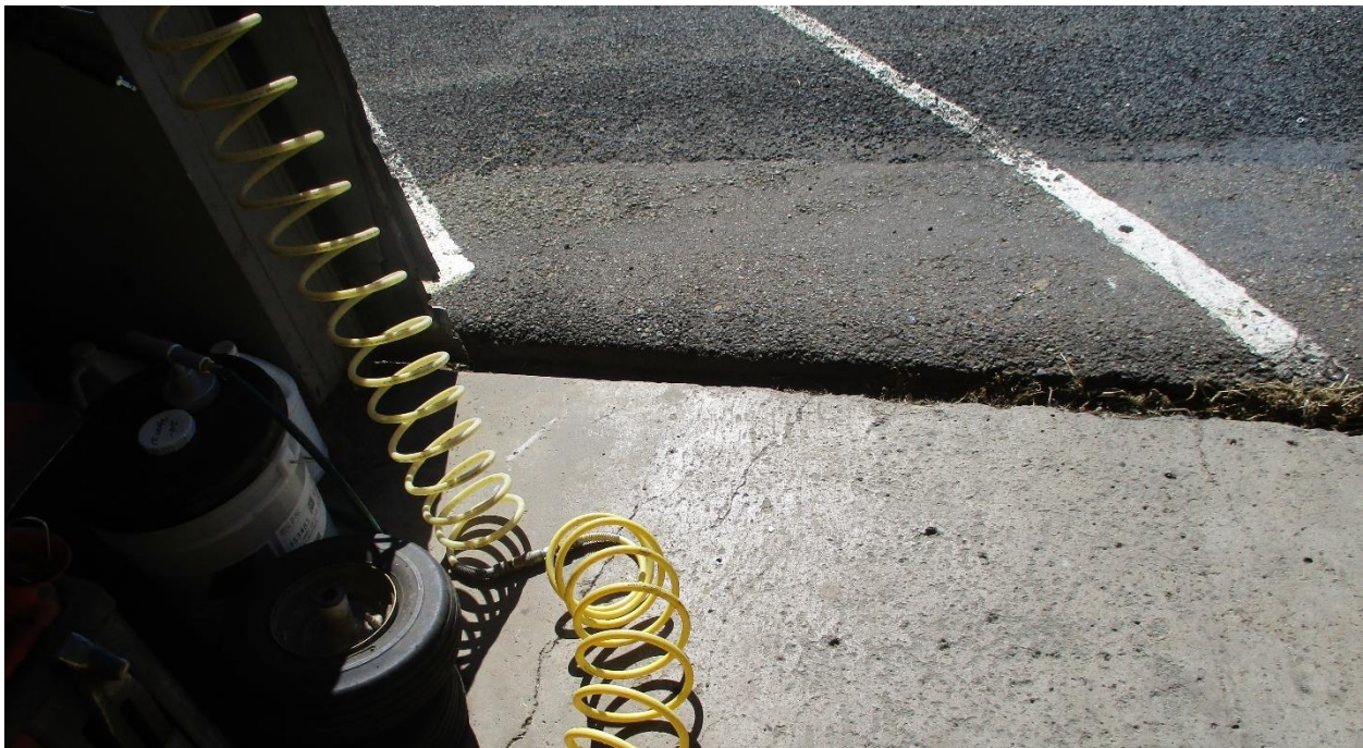
Figure 2.3. Example of Transition Between Asphalt and Concrete
