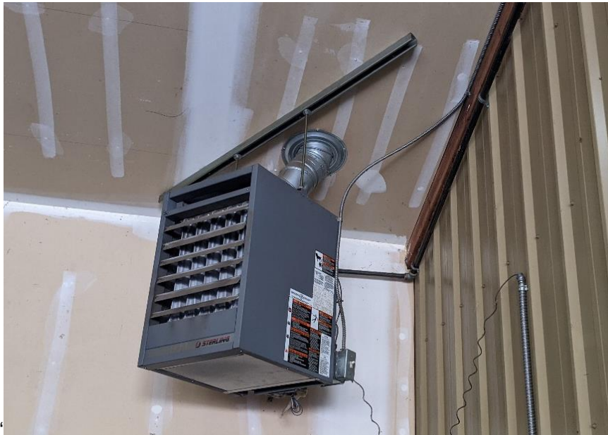
Figure 4.17. Building E Unit Heater
