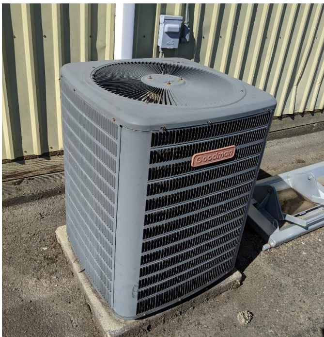
Figure 4.5. Building A Workshop Heat Pump
