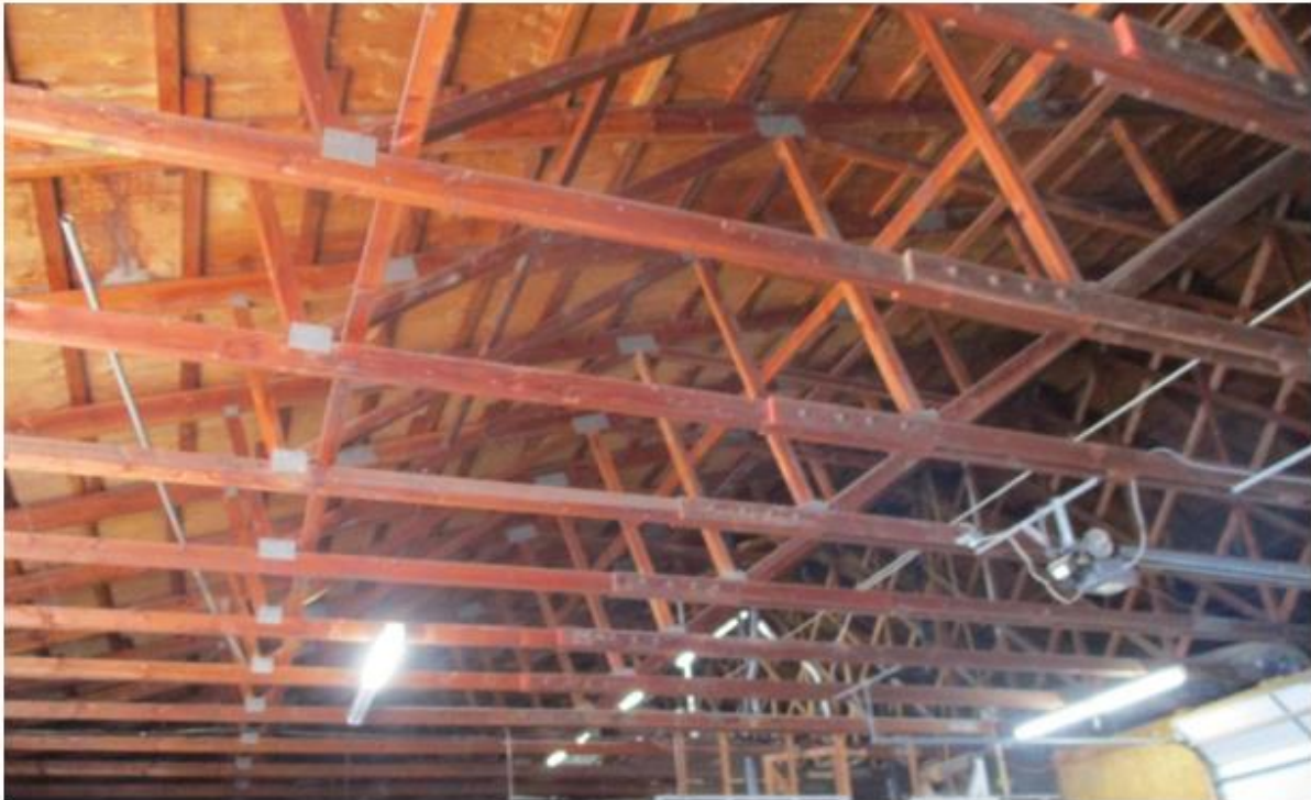
Figure 2.1. Wood Trusses Supporting Roof
