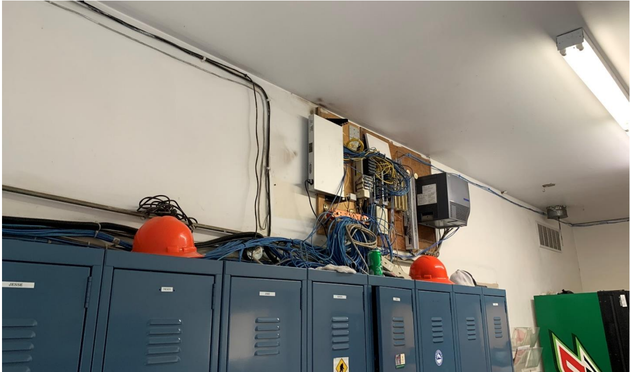
Figure 3.3. Exposed Communication Equipment
