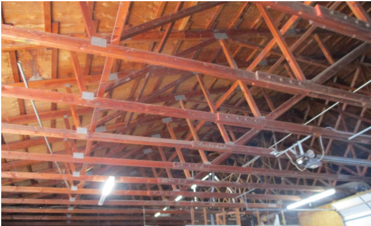
Figure 2.1. Wood Trusses Supporting Roof
