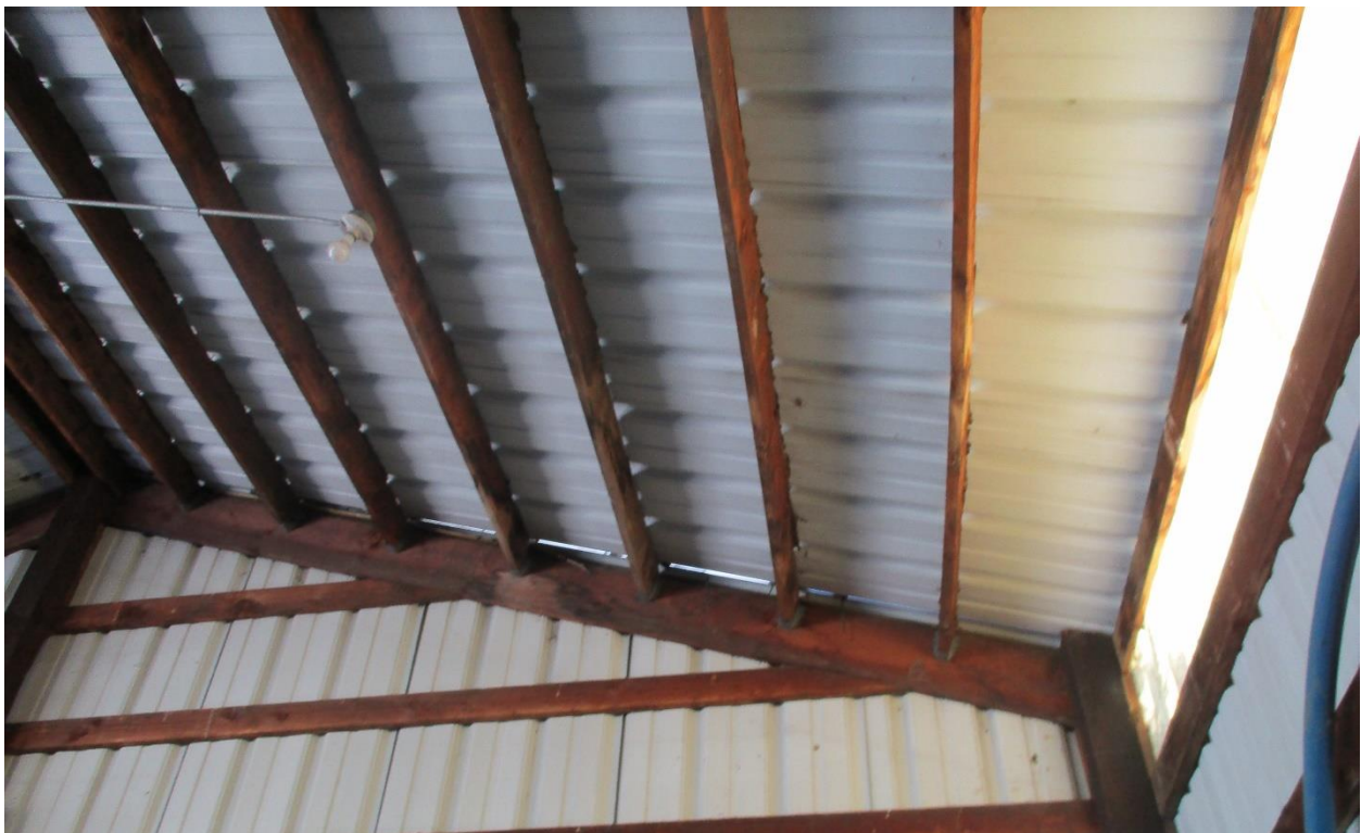
Figure 2.9. Gap at Edge of Roof
