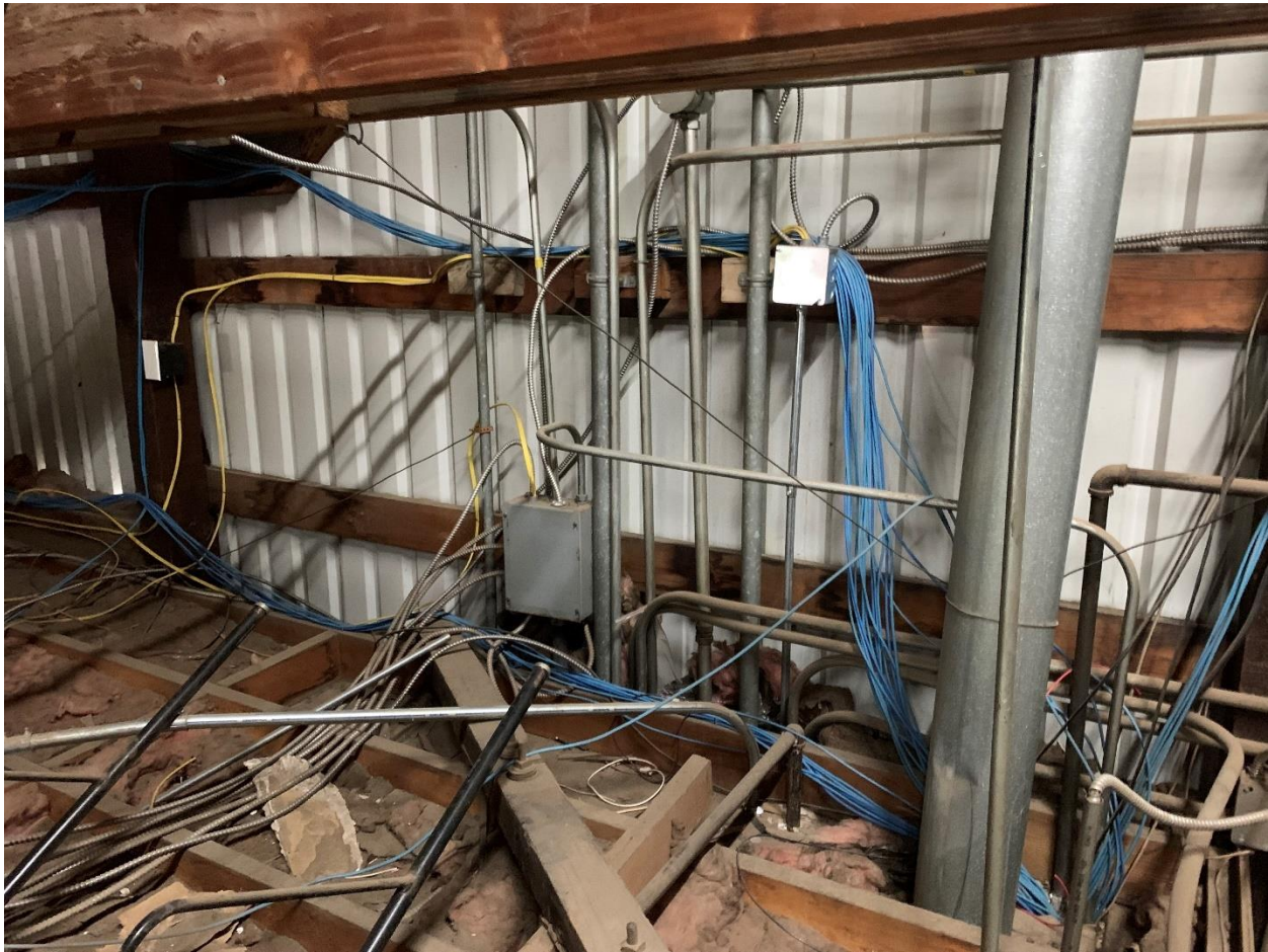
Figure 3.4. Communication Cables in Attic
