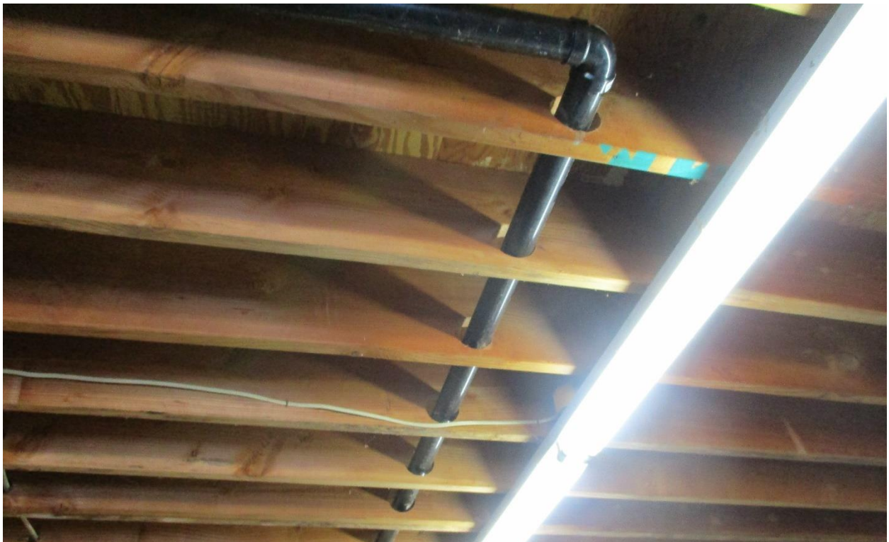
Figure 2.15. Holes Drilled in Joists
