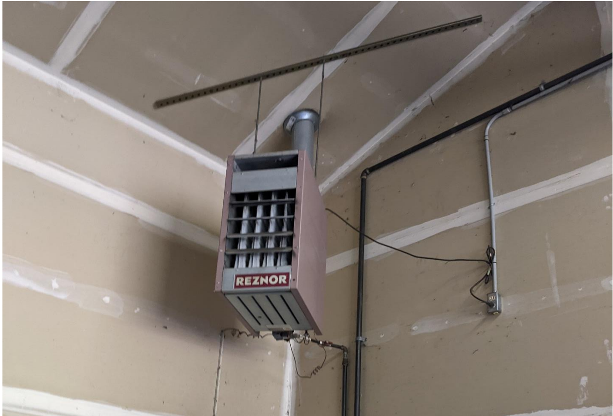
Figure 4.15. Building D Gas Unit Heater
