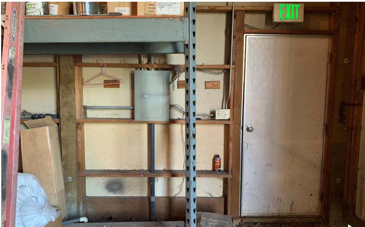
Figure 3.10. Metal Shelf in Front of Panel
