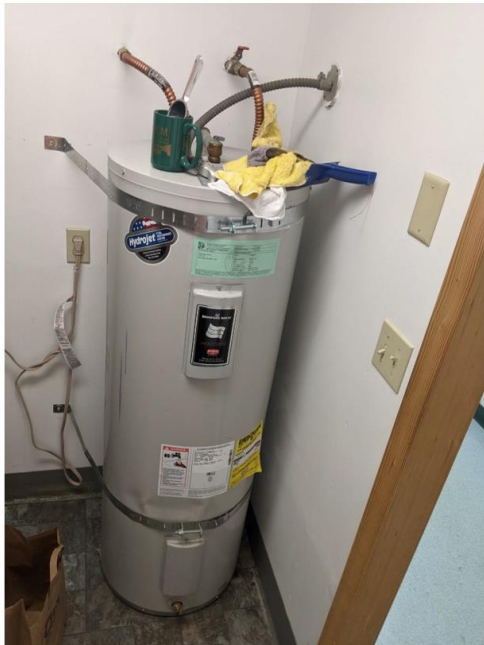
Figure 4.8. Building A Domestic Water Heater
