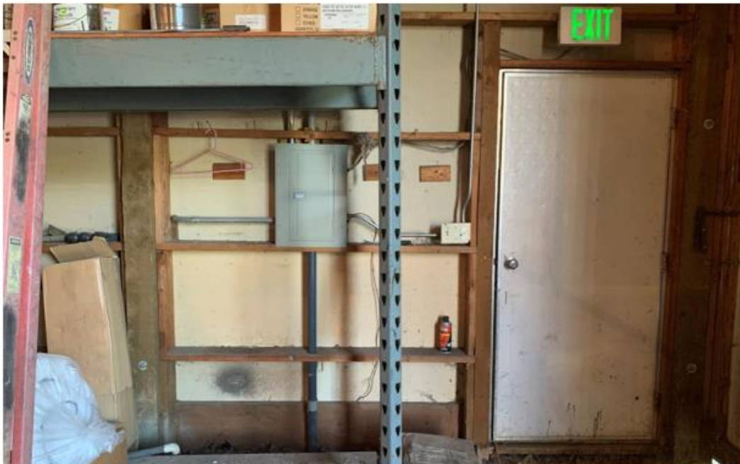
Figure 3.10. Metal Shelf in Front of Panel
