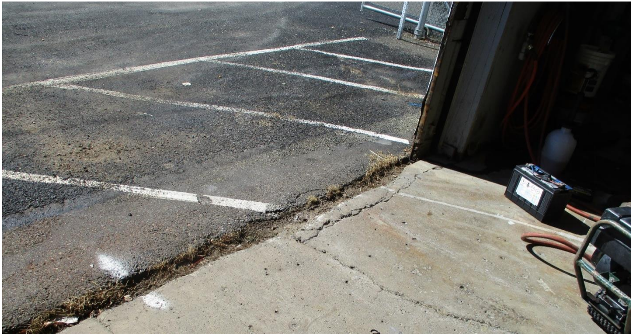
Figure 2.2. Example of Transition Between Asphalt and Concrete
