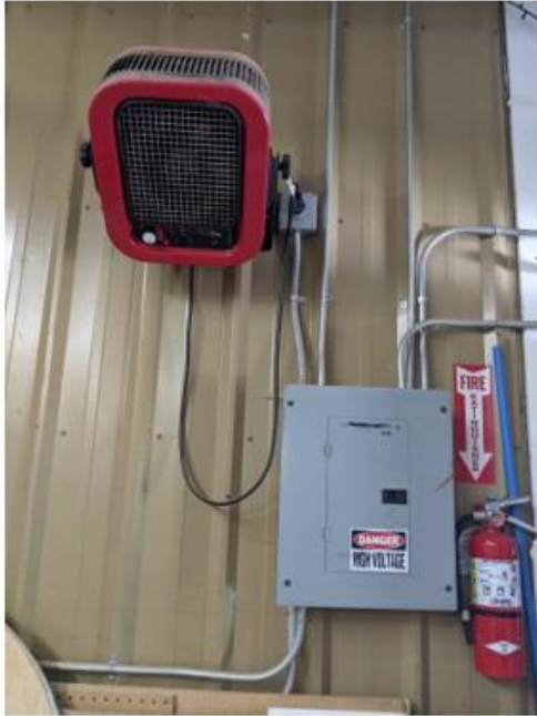
Figure 4.19. Building F Electric Unit Heater in Entry Area Shop
