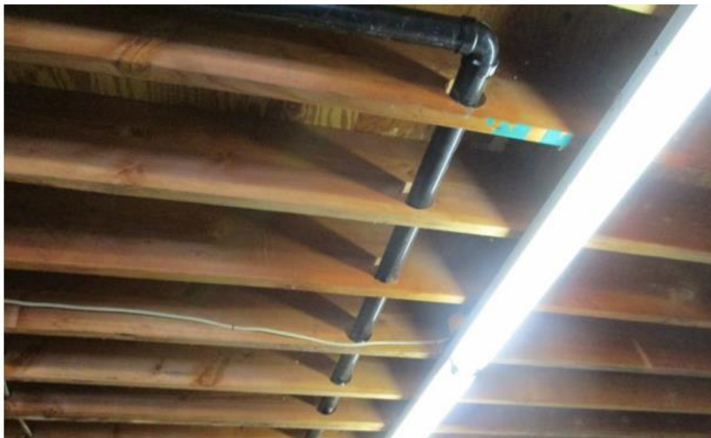
Figure 2.15. Holes Drilled in Joists
