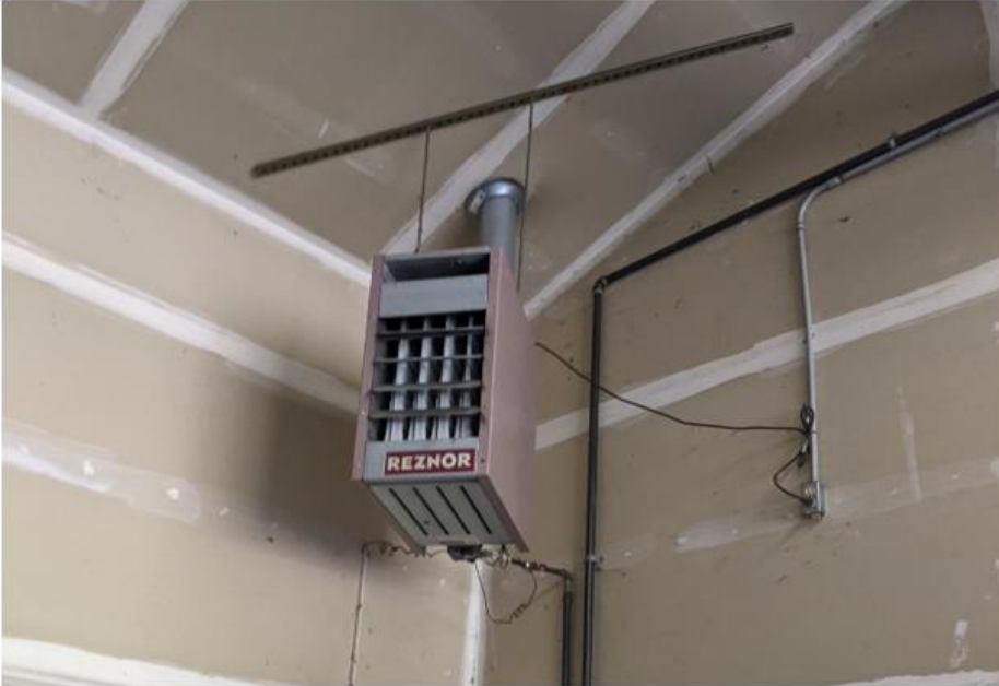
Figure 4.15. Building D Gas Unit Heater
