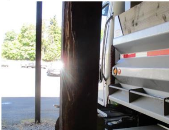
Figure 2.11. Column Damage
