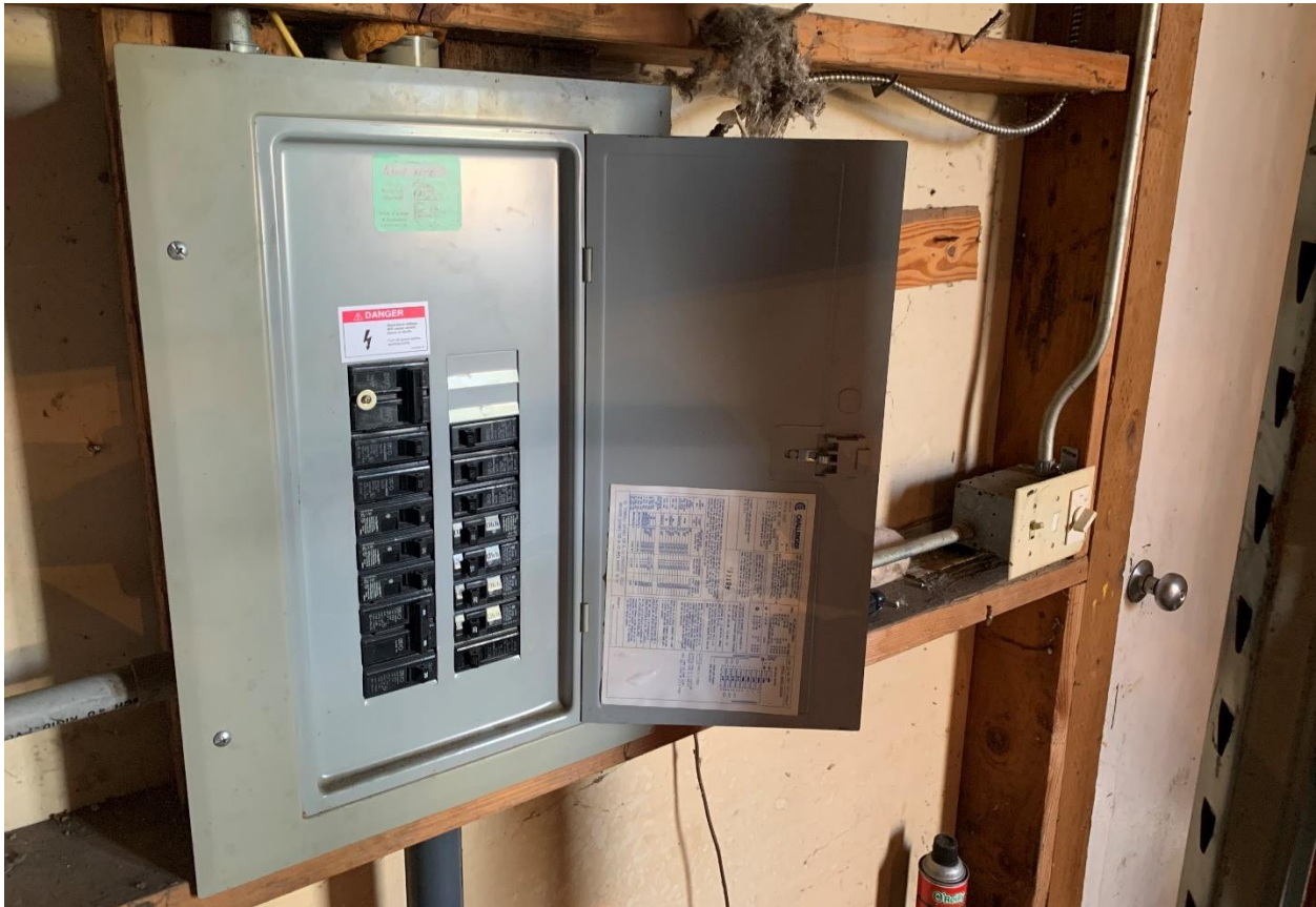
Figure 3.10. Metal Shelf in Front of Panel
