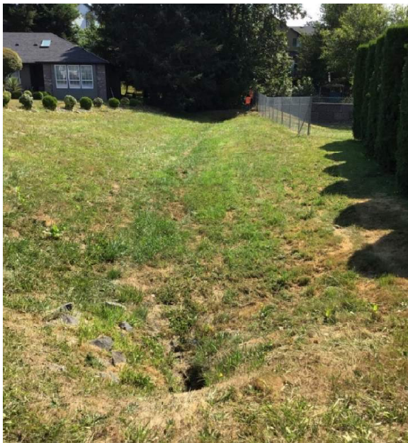
Biofiltration swale, looking East, site visit July 27, 2022.
