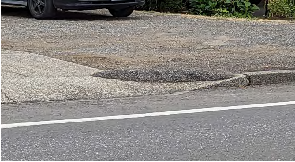
Residential homeowner created asphalt berm to divert flows away from driveway. Field photo dated September 13, 2023.
