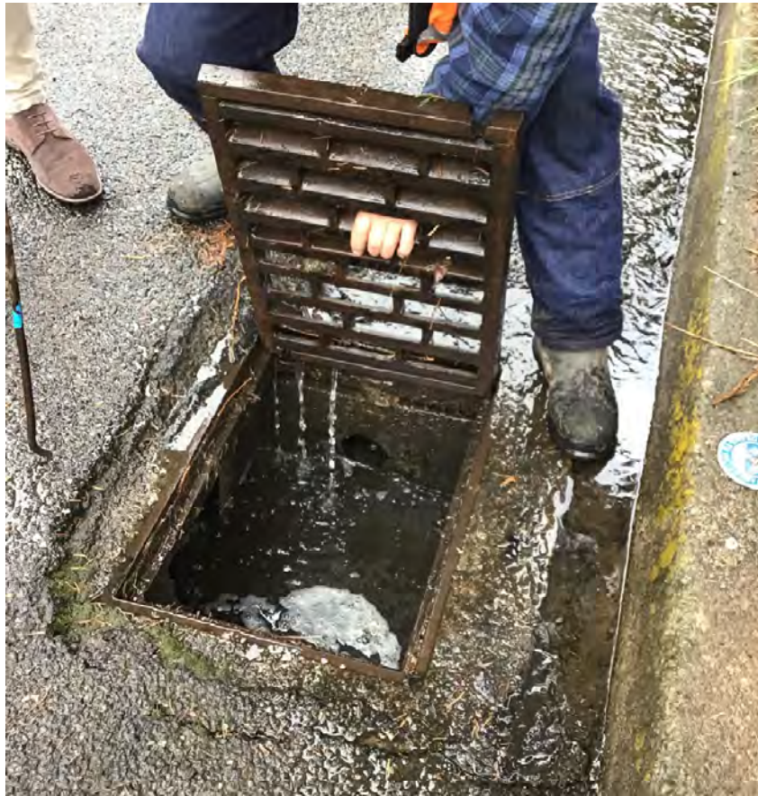
Looking in undersized catch basin on north side of Addy Street. Field photo date April 7, 2023.
